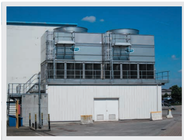
➤ High efficiency cooling tower
