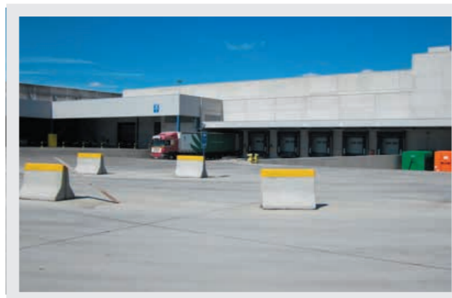
➤ New loading/unloading bays
